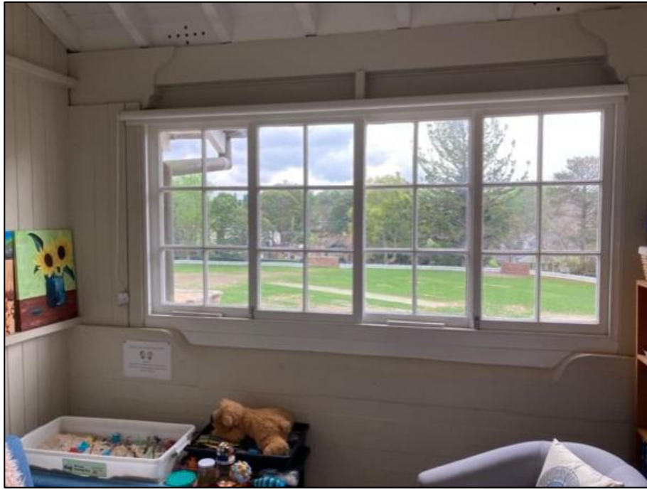
Figure 36: An example of an office on the first-floor within a later verandah enclosure. This glazing is proposed for removal with new full height glazing inserted to recreate the appearance of an open verandah.
