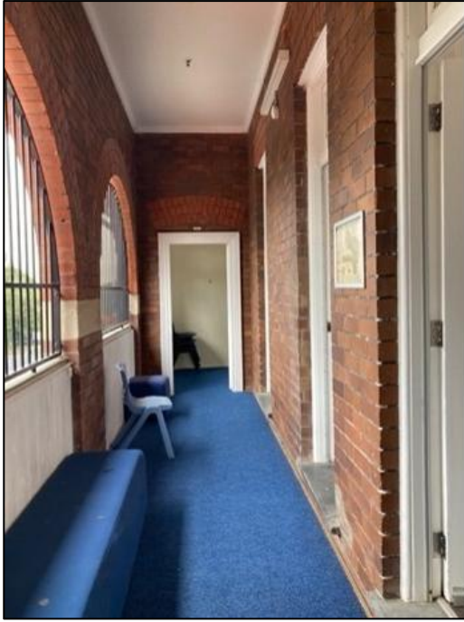
Figure 38: Semi-enclosed verandah on the southeast side of the building. Note the metal grilles to the left which will be removed and replaced with glazing and the timber balustrades retained and repaired.
