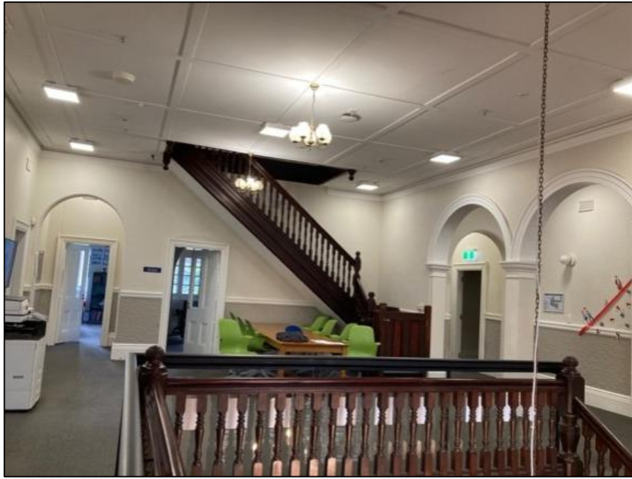
Figure 34: First-floor landing, looking towards stair to the attic. Note arched openings. The opening on the far left will be blocked by new full height glazing which will retain visibility of the arch while preventing access.
