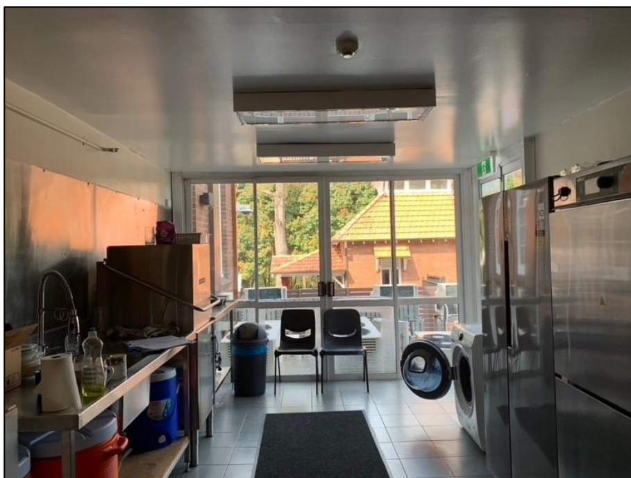
Figure 31: Kitchen on the ground-floor showing contemporary fit-out and finishes. This fit-out is proposed for removal and the room turned into a store. The contemporary glazing at the end will be replaced with new glazing above a brick cavity wall.
