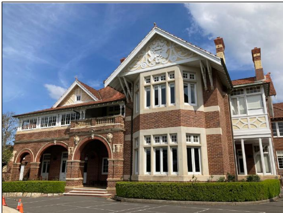
Figure 17: Front elevation. Note the partially enclosed first-floor verandah to the left. It is proposed to remove the multi-paned glazing and replace with new full height glazing suites.
